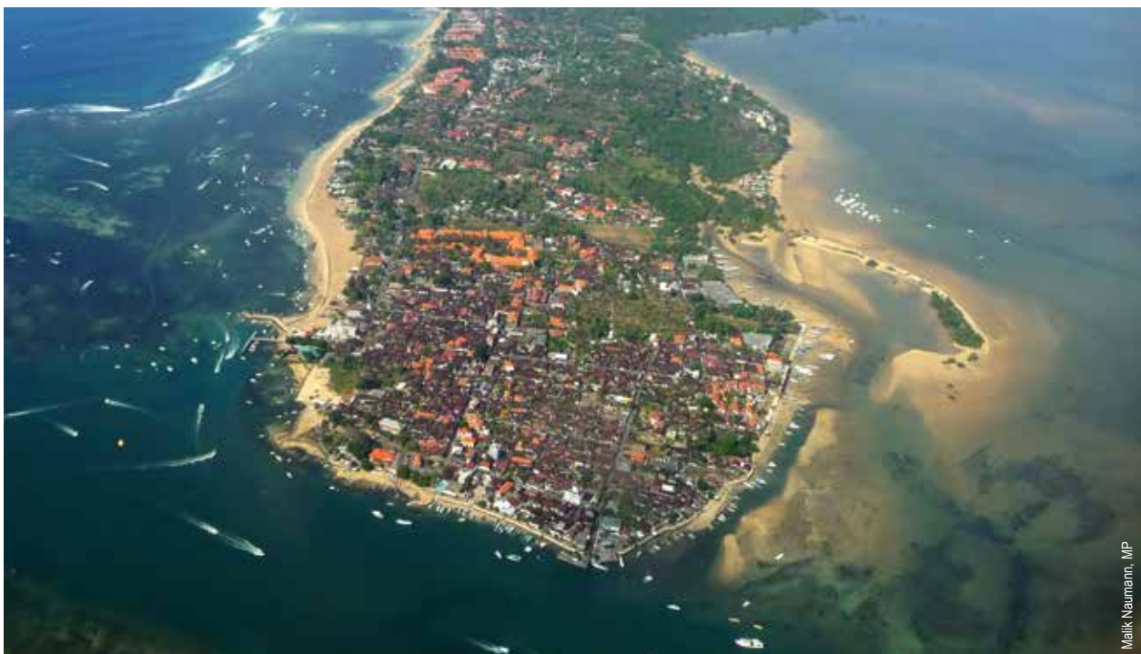
Pembangunan di wilayah pesisir, Nusa Dua, Bali, Indonesia. Building construction at Nusa Dua coastal area, Bali, Indonesia.
